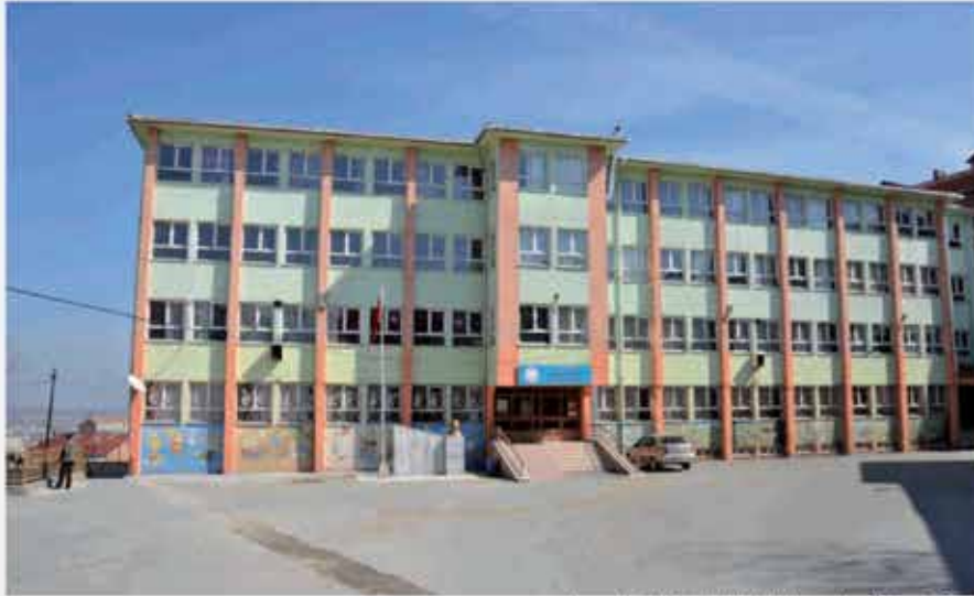
Arnavutköy İlköğretim Okulu / Arnavutköy Primary School
